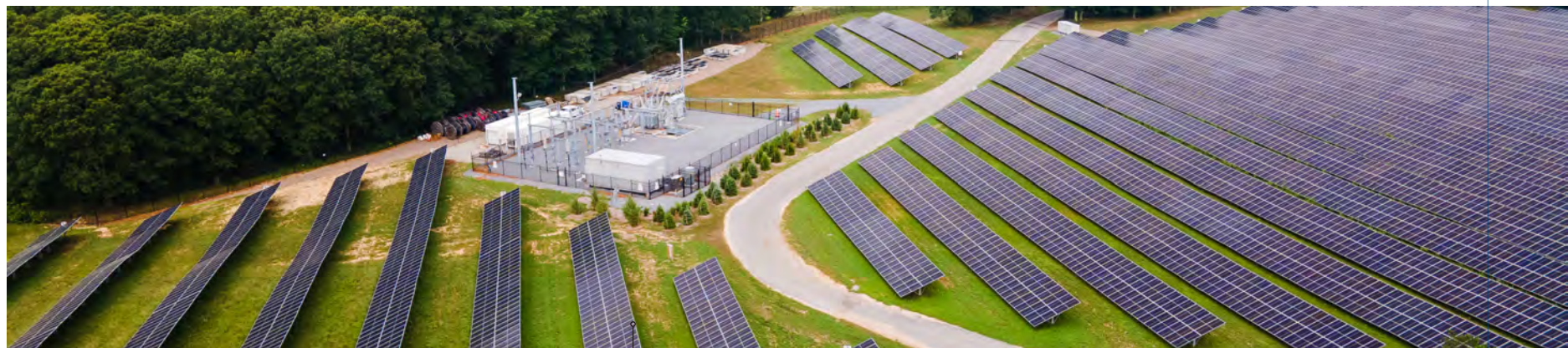
Calverton Solar Energy Center | Calverton, New York
