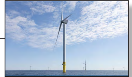
South Fork Wind Farm (132 MW) 35 miles off Montauk, New York
