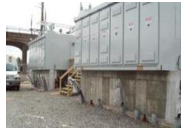
Figure 6. Far Rockaway (left) and Arvene (right) substations after implementation of storm hardening projects.
