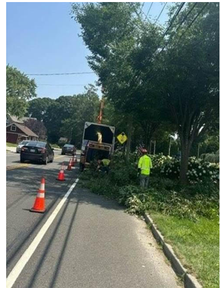
Figure 9. Completion of pruning to create a buffer between the power lines and nearby trees, reducing outage threats.
