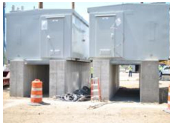
Figure 6. Far Rockaway (left) and Arvene (right) substations after implementation of storm hardening projects.
