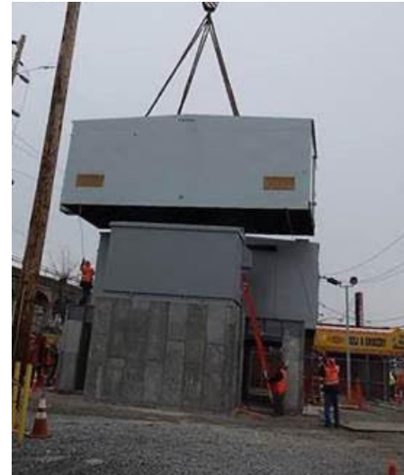
Figure 8. Installing an elevated switchgear at the Arverne Substation.
