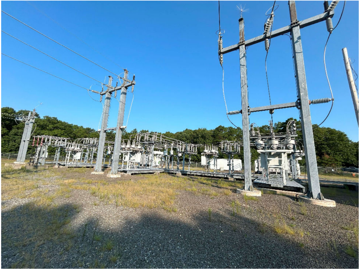
Figure 4-3: Overall Condition of 8WF William Floyd Substation
