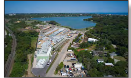
Montauk Energy Storage Center (5 MW) Montauk, New York
