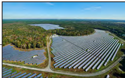
Long Island Solar Farm (32 MW) Upton, New York
